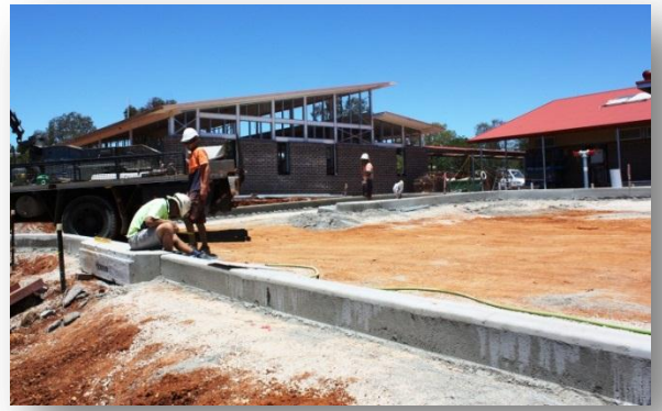
Brickwork outside of Block D (pool area)
