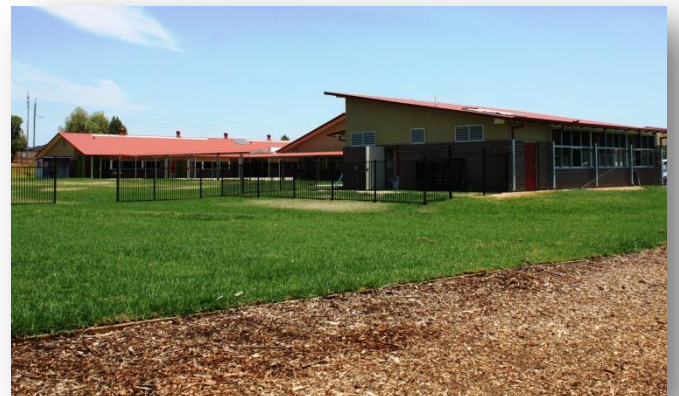
Near completion – view from Lincoln street
