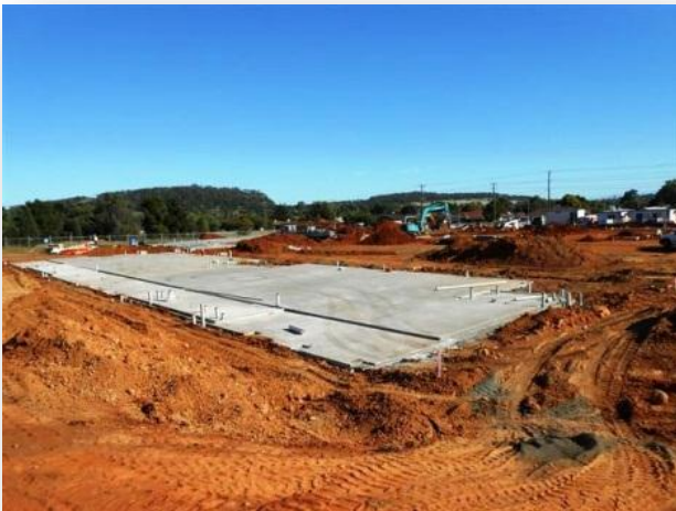
Laying the foundations for the admin building
