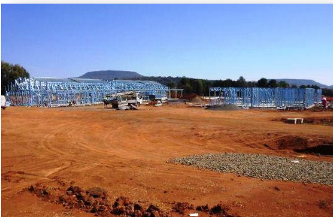
Framework for Block A (admin) and Block C (classrooms)
